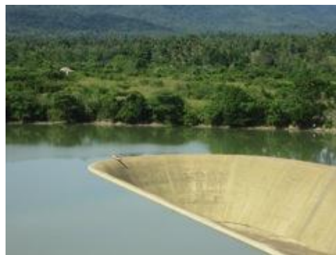
Figure 3: Malinao Dam in Pilar, Bohol
